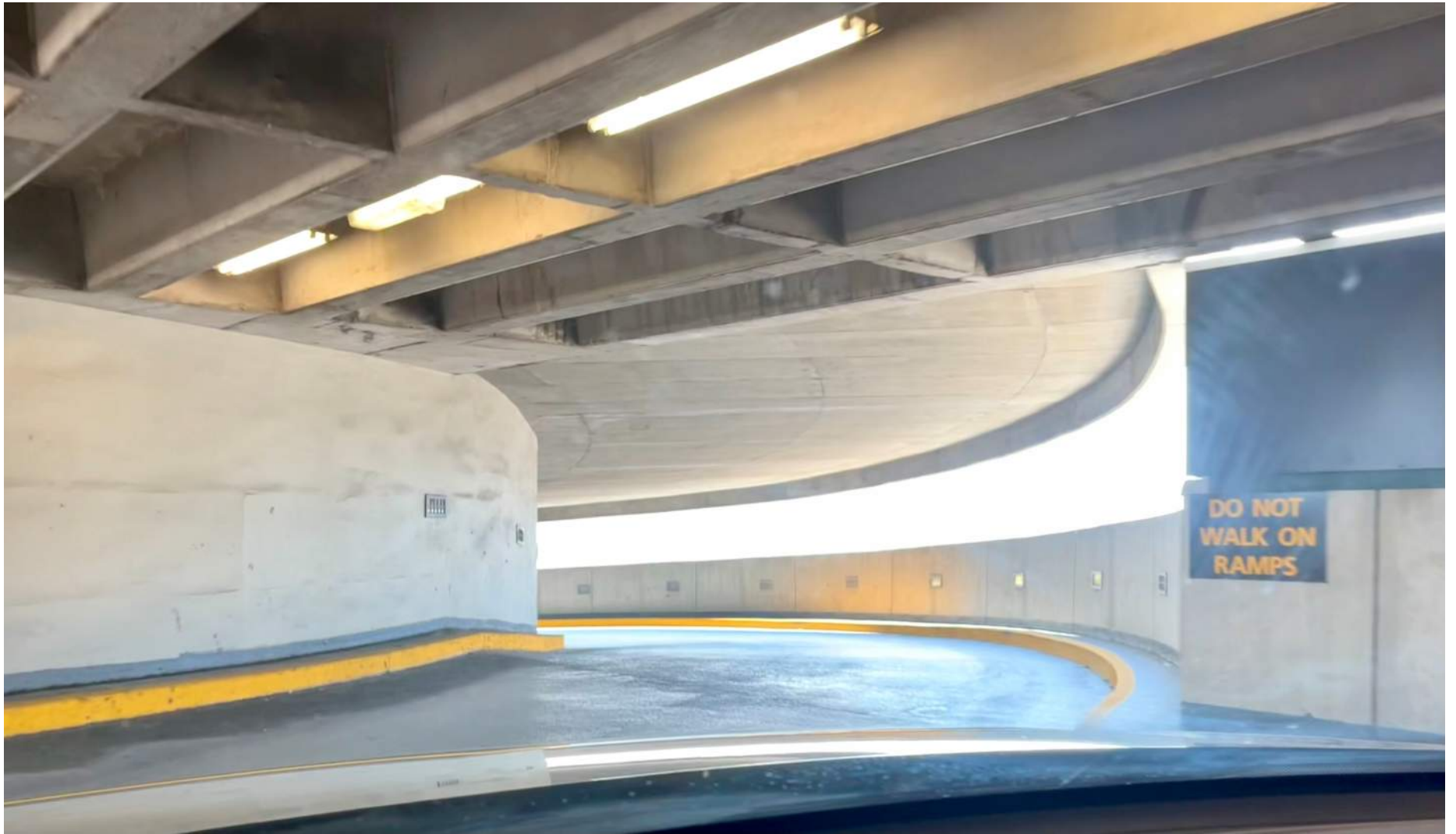
Example of a vehicle only ramp with signage against pedestrians using ramp.
